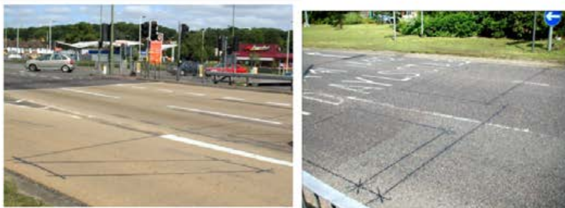
Figura 14 – Bucle inductive instalate in asfalt (exemplu)
